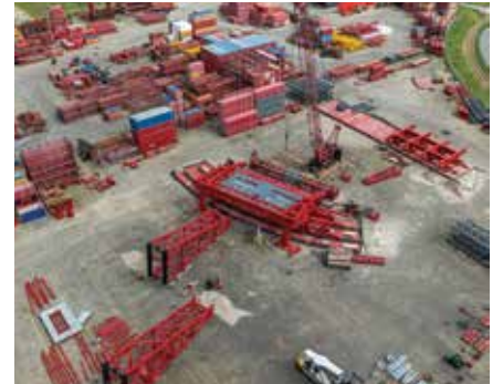
The slewing track takes shape
