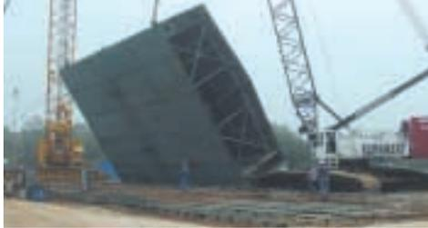
MASTER BOAT Builders Inc of Coden, Alabama, US, relied on the powers of Barnhart Crane & Rigging to roll three massive components to be used in the construction of a crew boat set for duty in the offshore industry. Barnhart called on two of its Demag crawler cranes for the job, a 544 tonne capacity CC2600 and a 299 tonne capacity CC2000, to "bookend" each of the three sections of the boat, the heaviest of which weighed 290 tonnes. A fourth component weighing 118 tonnes was then set in place.
