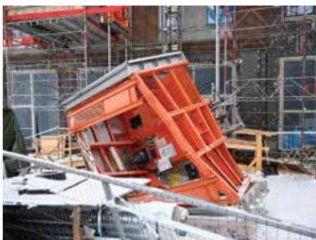
Five occupants in this hoist car died when it crashed to ground from a height of around 20 metres
