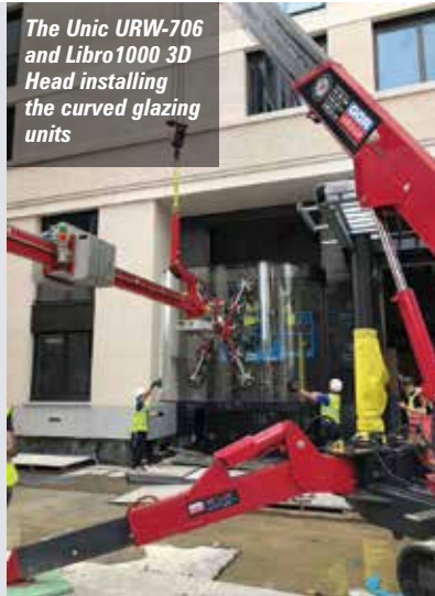
The 3D head provided 60 degree powered tilt, and 40 degrees left and right of centre slewing as well as powered 95 degree rotation
