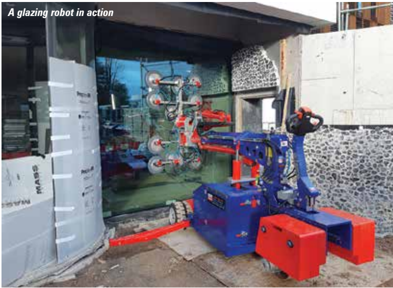
Most glazing robots have no outriggers and a basic three wheel chassis
