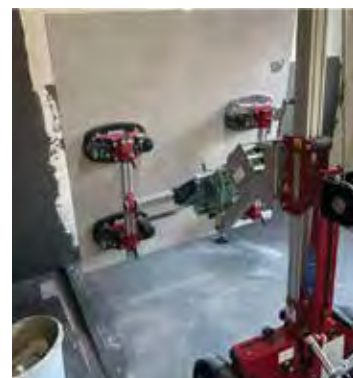
A glazing robot installing large ceramic tiles indoors
