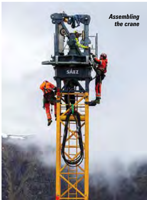
The tower crane almost fully assembled
