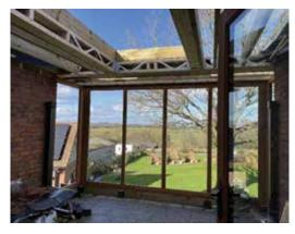
The HSE investigation found no external scaffold had been installed to provide safe access, no internal measures were in place to prevent falls, while the work was not properly planned or with suitable safety instructions provided to those working on the job.
