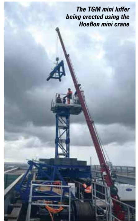
The TGM erecting the Comansa flat top
