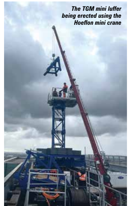
The TGM erecting the Comansa flat top
