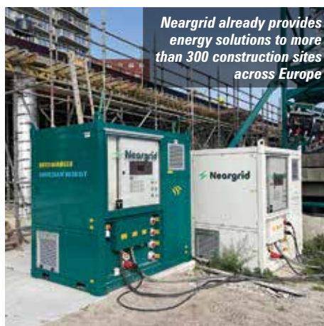
Bowmer + Kirkland was an early adopter in replacing diesel generators with energy storage systems to power tower cranes on site
