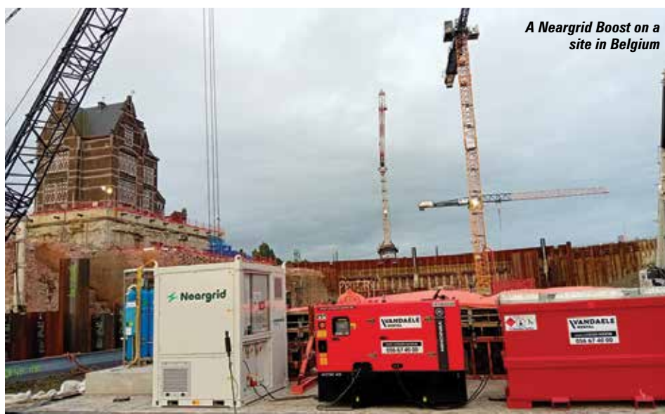
A battery storage system powering mastclimbers and hoists
