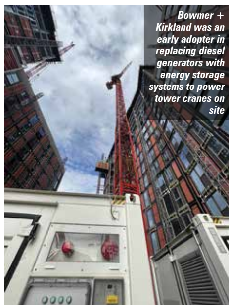
A battery storage system powering mastclimbers and hoists
