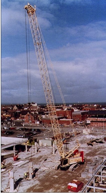
The new Liebherr LR1100 can be assembled within an hour
