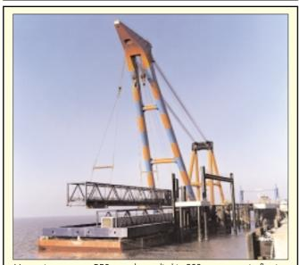
Norwegian company DDB recently supplied its 900 tonne capacity floating crane Samson to lift this 250 tonne steel linkspan bridge into position at the Port of Hull. The load is one of two passenger and vehicle linkspans which will connect the terminal building to the new P&O super-cruise ferries which come into service later this month. The bridge is part of a major £10 million upgrade undertaken by Kier Northern for Associated British Ports. The project was completed in mid-April.
