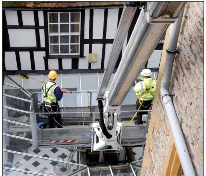
One of the trickiest areas to reach was an internal glazed-in courtyard - the Eagle's 17m jib and built-in pressure washer proved ideal.
