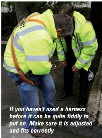
*If you haven't used a harness before it can be quite fiddly to put on. Make sure it is adjusted and fits correctly*
